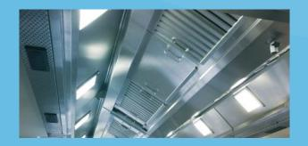
In island applications, surface-mounted air curtains are effective in reducing exhaust requirements. An air curtain is an invisible wall created to capture the plume, transport it into the hood cavity and provide resistance to cross-draughts.
