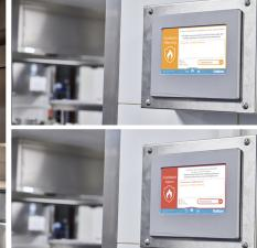
**Stage 1 alarm** - A warning is displayed on Halton Touch Screen. It is relayed with light signal and buzzer fiited on the front of the hoods.
