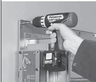
**7** When the power is off, the electric actuator can be tested manually by means of a hexagonal spanner (included in the delivery).
