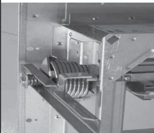
**2** In installation of the fire damper on panel walls, a steel frame or a wooden joist must be mounted on the edges of the opening, supported against the wall joists.
