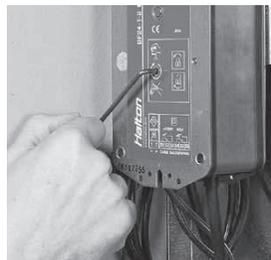
**9.** The electric actuator fuse can be tested when the power is on, by means of the fuse switch.
