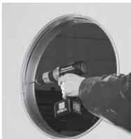
**5.** Centre the fire damper in the middle of the installation hole, and fix on a lightweight wall with steel screws (e.g., 6.5 x 50) or on a concrete and masonry wall or plate with an expansion anchor – e.g., M8 x 50 by the flange. Ensure the correct operation of the product before grouting.
