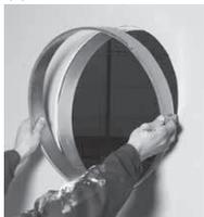
**4. Panel wall:** Fasten the installation frames together with screws or rivets, ensuring that they are simultaneously fixed to the steel frame or the wooden joist.
