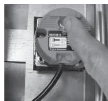
**10. Manual actuator:** Test the operation by freeing the lock of the handle. Lift the locking pin (with black knob) up, and turn 90 degrees by the handle. If the setting fails, the released fuse must be replaced. Simultaneously, the electrical and mechanical operation of the micro switches, which are available as accessories, should be tested.
