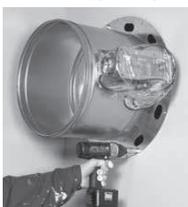
**6.** Cover the product and actuator while grouting. Grouting and sealing will be performed through the entire thickness of the wall with fine-grained concrete or fire prevention mastic, such as GBG (from Palokatkomiehiet Oy), CP 637 (Hilti), or Sealfire W1000 (Würth).
