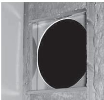
**2. Panel wall:** Fill the corners with a mineral wool that corresponds to the insulation of the wall. The wool must reach the round installation frame along its entire perimeter.
