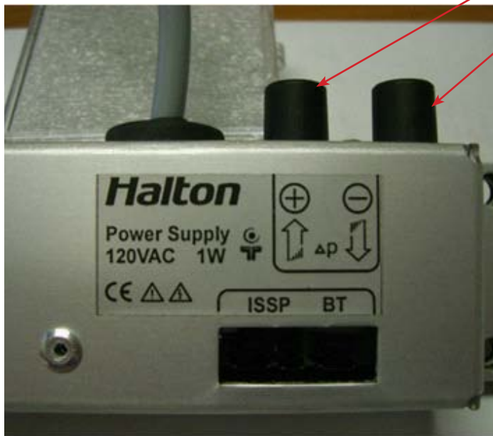
Photo 2 – AccuFlow Pressure Taps
