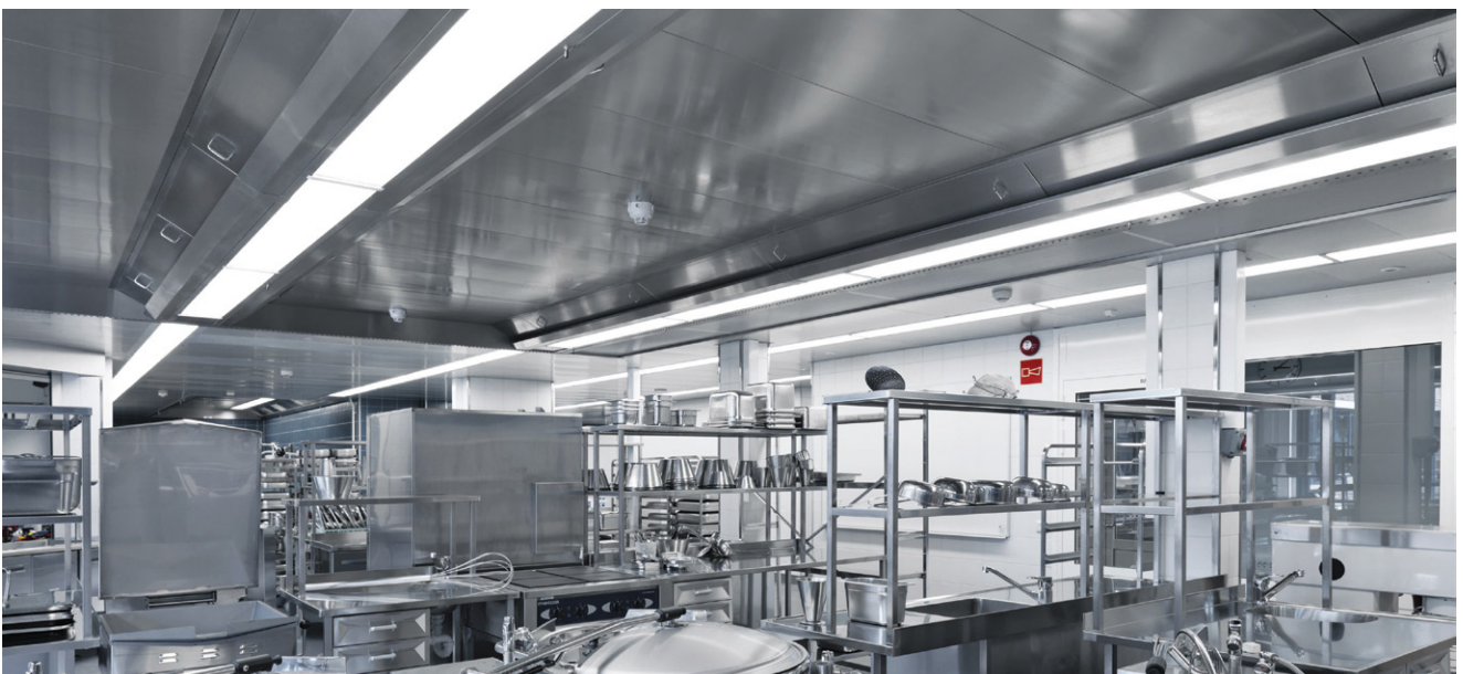
Kotka central kitchen (Kotka, Finland)
